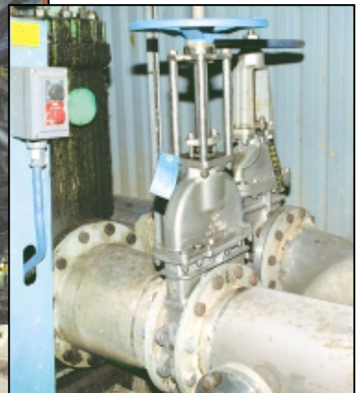
Filter isolation installation.
